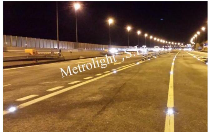
The "METROLIGHT ML-ITL" induction road stud is designed with a degree of protection IP68 and IK8 - IK10 with defence accessory.
